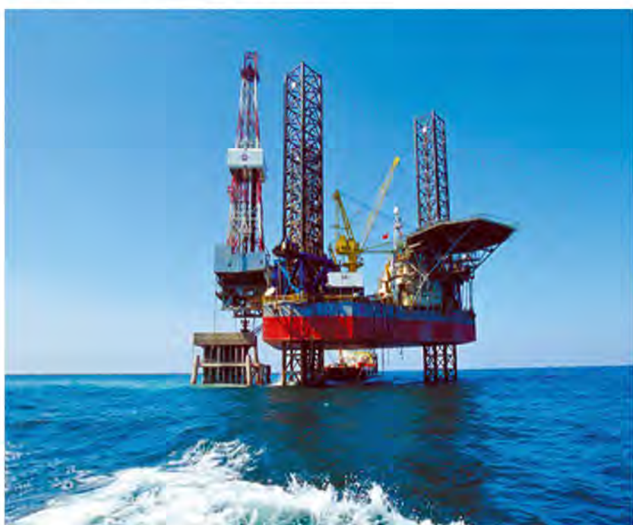
An offshore oil and gas platform (Courtesy of/www.nrgedge.net)
